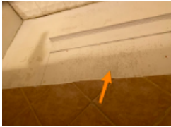
Fungal growth in bathroom, due to improper ventilation
